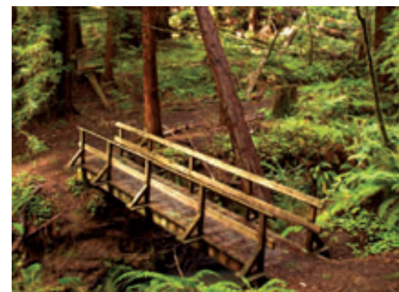
Bridge access over Butano Creek
