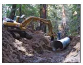
Placing new road culvert designed to withstand a 100 year storm event.
