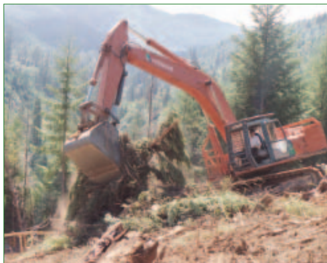
Excavators and bulldozers work in tandem to remove logging roads. Photo by League Staff
