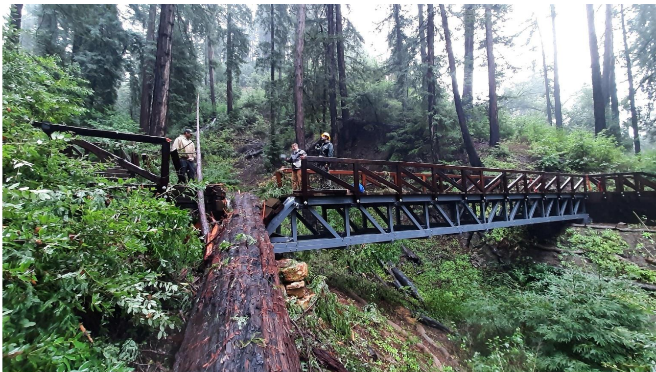
The Pfeiffer Falls Trail bridge was damaged by a fallen redwood tree in 2023, leading to a temporary trail closure. Photo from California State Parks
